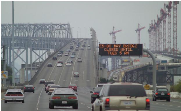
Bay Bridge I-80 westbound traffic with a CMS indicating extended bridge closure for construction.
