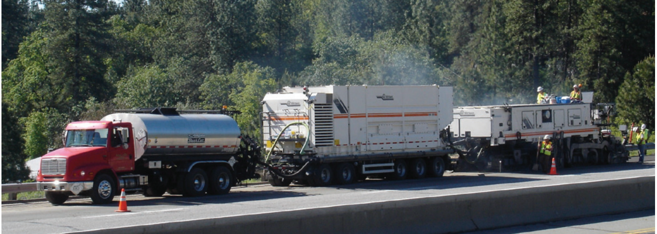
Cold-in-place recycling train.
