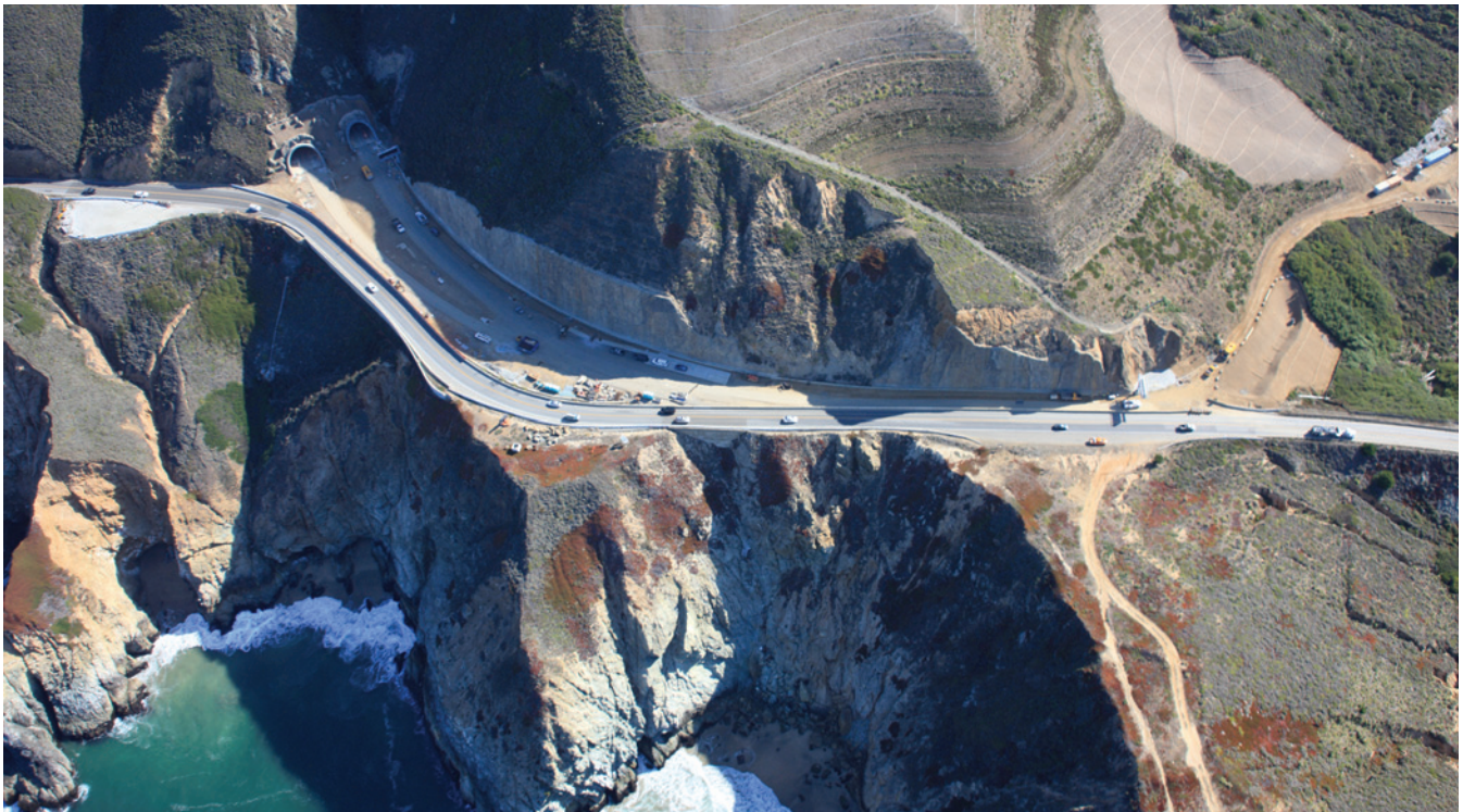
Aerial view of the south portal and roadway of the Devil's Slide Tunnel.
